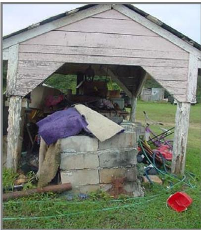
Unused water wells that are not properly abandoned leave open holes in the ground. These holes are dangerous. People (especially children), pets, and wild animals can get hurt or trapped after falling into an abandoned well. These holes serve as direct channels for contamination into Georgia's groundwater. They allow chemicals and bacteria from the surface environment to pass straight through to a drinking water source used by many people.
